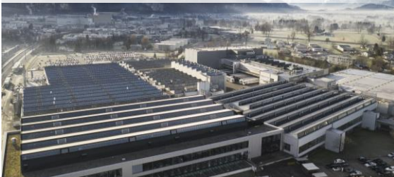
Lighting plant, Dornbirn (AT)
