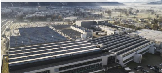
Lighting plant, Dornbirn (AT)
